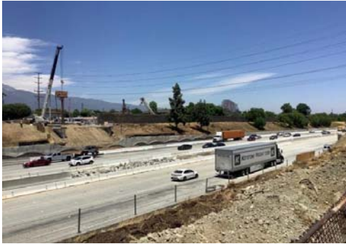
Photo: San Bernardino County Transportation Agency
